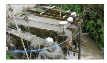
raised or diverted channel, which must create an elevation drop (head) of at least 1.5 m. This type of installation is usually found in the northern part of Laos where the landscape is hillier, which provides high head. Standing installations also provide more stable electricity due to more effective control of water flow to the pico turbine via the intake channel.
