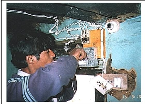
Figure 15-1 Installation of domestic wiring circuit (Nepal)
