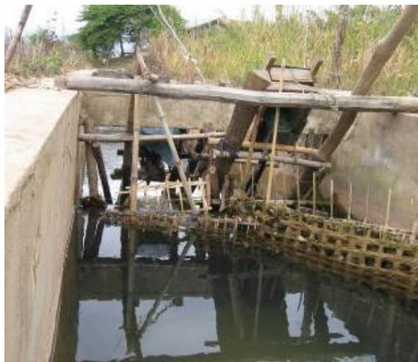
Figure 18 - Pico-hydro unit in irrigation channel in Moh village
