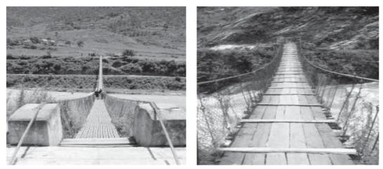
Wooden walkway deck need changing every three to four years. Galvanized steel walkway deck is relatively 'maintenance-free'
