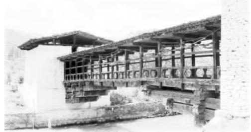
A traditional Bazaam bridge - roofed wooden cantilever bridge, Bhutan
