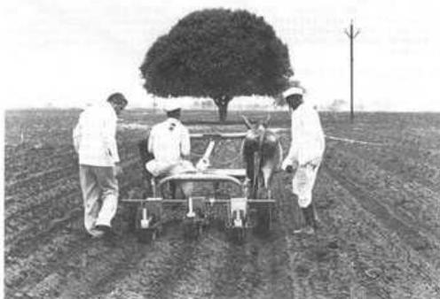
Plate 5.7 Trials at ICRISAT of a 3-row planter on broad beds (ICRISAT)
