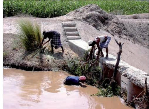
Blocking scour sluice on a modernised spate irrigation system in Yemen. (spate-irrigation.org)
