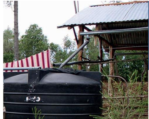
Semi-circular guttering with "circular" extended guttering. (C. Studer)
