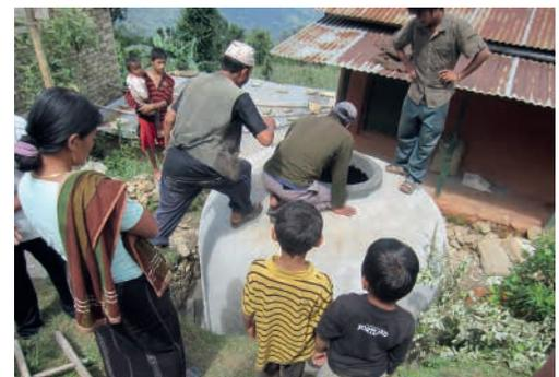
A rainwater storage tank constructed by householders in Nepal. (RAIN)
