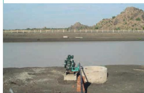
Excavated pond (improved *hafir* system) with water pump and sedimentation tank. (Ministries of Water Resources and Irrigation of Sudan and South Sudan, 2009)
