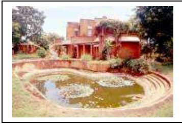
Biological wastewater treatment
