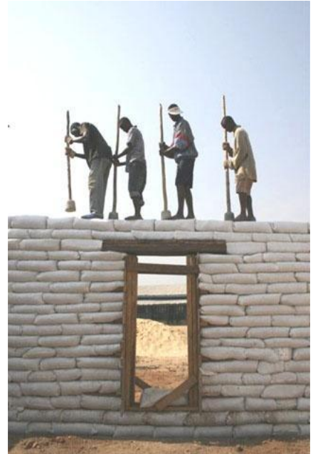
RIGHT: TAMPING AN EARTHBAG SCHOOL WALL IN SIERRA LEONE
