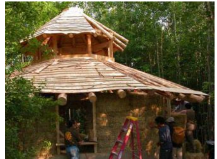
RIGHT: AN OCTAGONAL POLE ROOF WITH A CUPOLA
