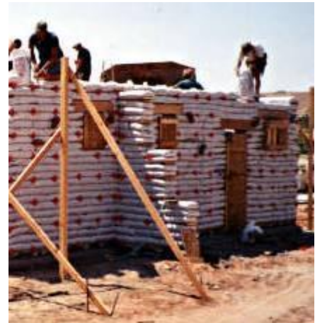
RIGHT: STEPPED BUTTRESSES IN UTAH
