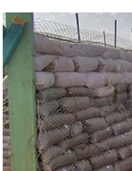
LEFT: MESH AND REBARS STRENGTHEN EARTHBAG
