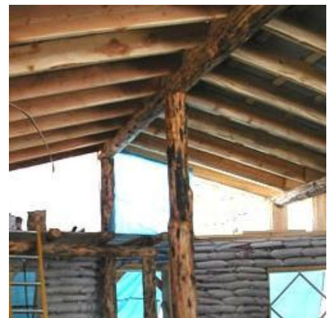
ABOVE: GABLE FRAMING ABOVE EARTH BAG WALLS
