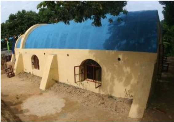
LEFT: FERROCEMENT VAULT ON A PHILIPPINE EARTH BAG SCHOOL
