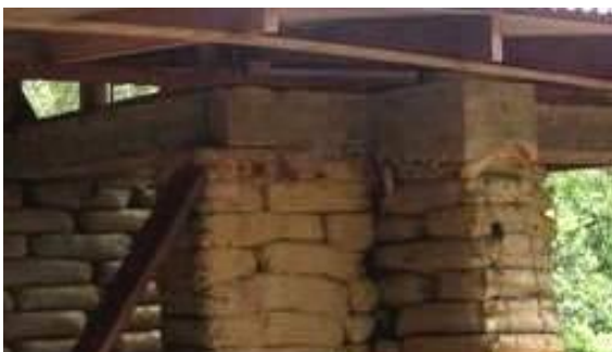
LEFT: REINFORCED CONCRETE BOND BEAM
