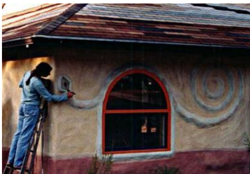
BELOW: DECORATED EARTHEN PLASTER ON AN EARTHBAG BUILDING
