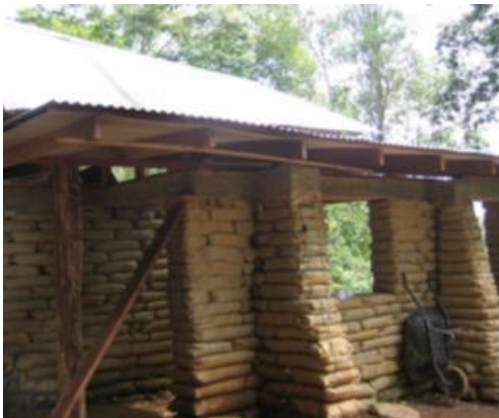
BELOW: SLOPING BUTTRESSES IN COSTA RICA
