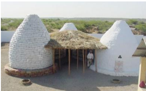
ABOVE: THREE DOMES SUPPORT A CENTRAL ROOF
