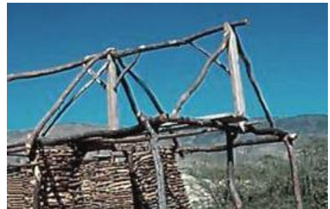
RIGHT: ROOF FRAMING FOR HAITIAN KAY
