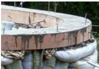
LEFT: CURVED REINFORCED CONCRETE BOND BEAM
