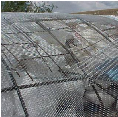
BELOW LEFT: MESH AND REBAR STRUCTURE
