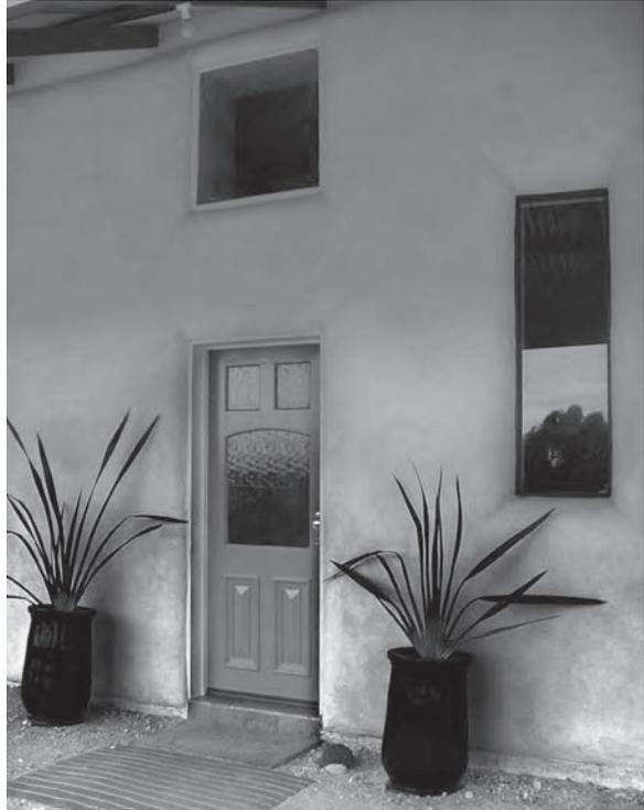
**Figure 5.4** Completed door and window buck made from 190 × 45 timber
