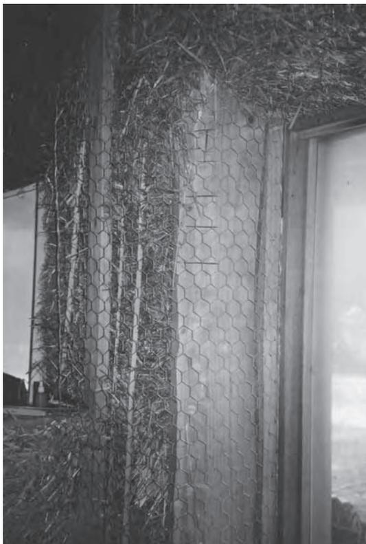
**Figure 5.20** Wire over 290 × 45 door buck stile to facilitate rounded render at the door opening
