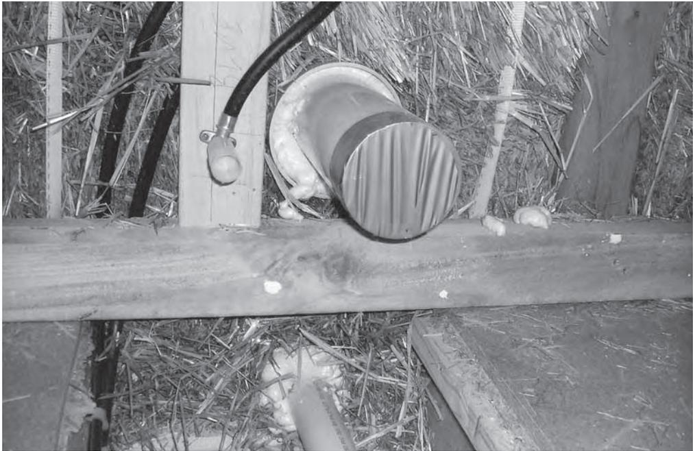
**Figure 13.1** 100 mm sewer pipe through 150 mm pipe with expanding foam sealant
