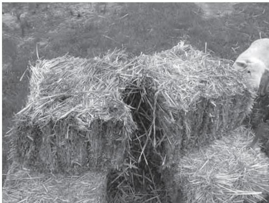
**Figure 4.16** The original ties on the bale are cut and the bale is separated into the two new lengths
