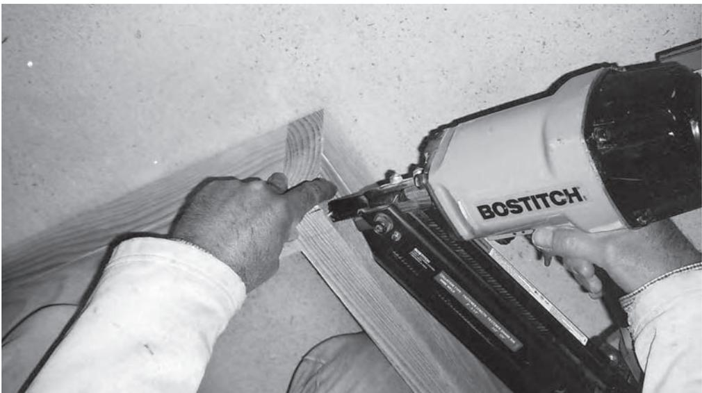
**Figure 14.8** Fix the head of the door jamb to the stiles
