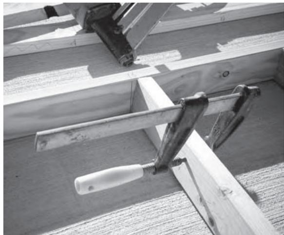
**Figure 6.11** Use a clamp to straighten twisted studs prior to installation
