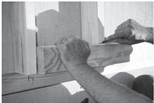
**Figure 6.15** Marking the stud with the depth of the lintel to be fitted
