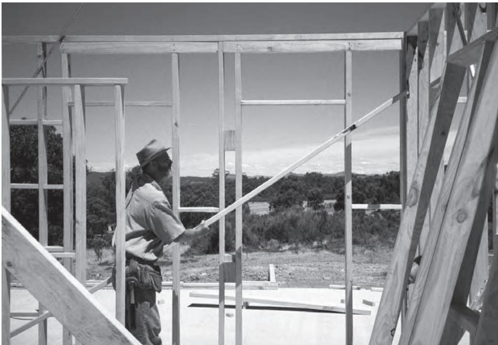
**Figure 6.18** Force wall frames into a vertical position using 90 × 35 pine
