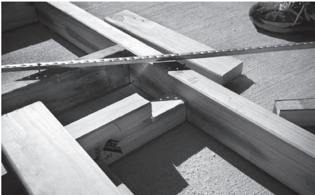
**Figure 6.16** Completed checkout in the stud ready for the installation of the lintel
