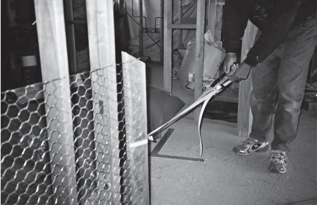
**Figure 6.20** Tightening the wire netting across the face of the wall using the compression strap tensioning tool
