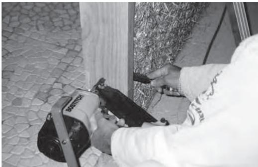
**Figure 14.9** Fix the bottom of the jamb stile to the frame
