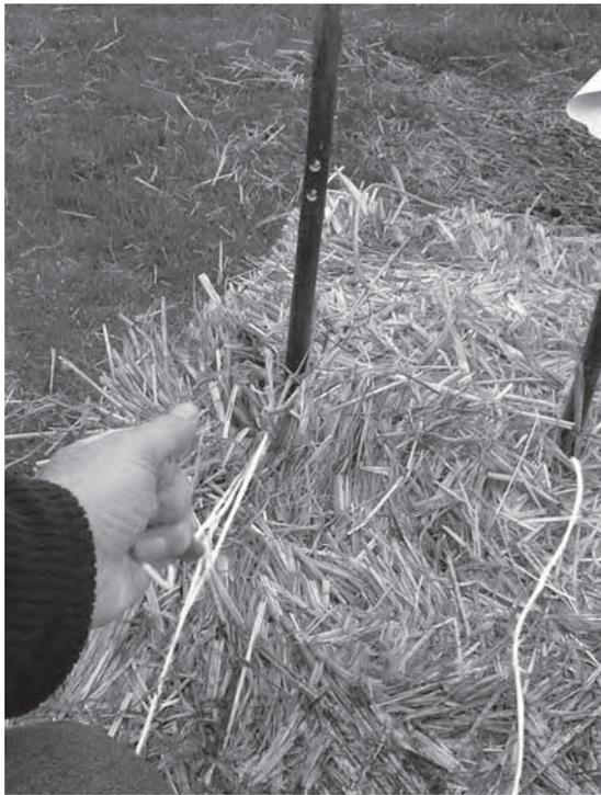
**Figure 4.15** The twine is tied around the new length bales
