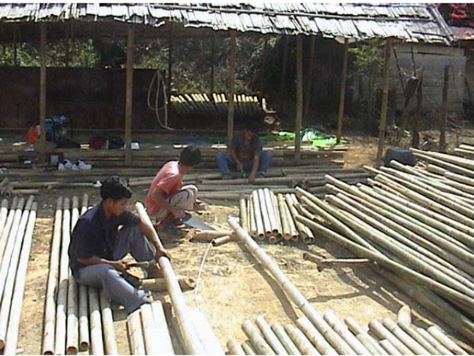
*Bamboo culms being sawed to size for use in housing*
