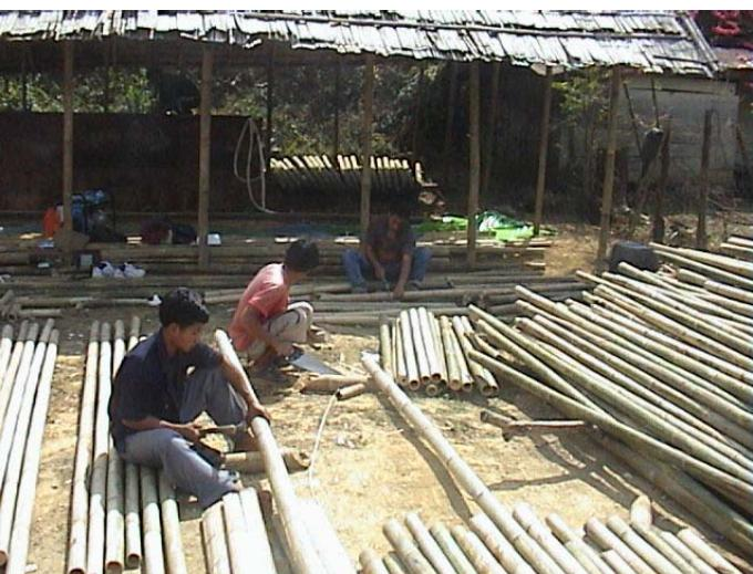
Bamboo culms being sawed to size for use in housing
