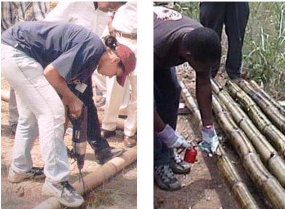
Pictures 1-2: Drilling and Injecting Creosote Oil
