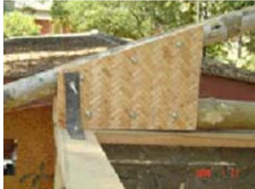
Pictures 25-26: Truss hanging and fixing
