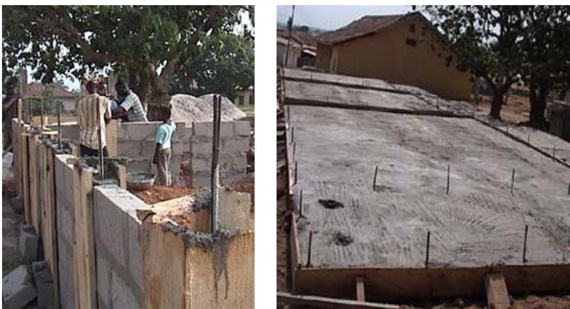
Picture 11-12: Foundation column and ground slab
