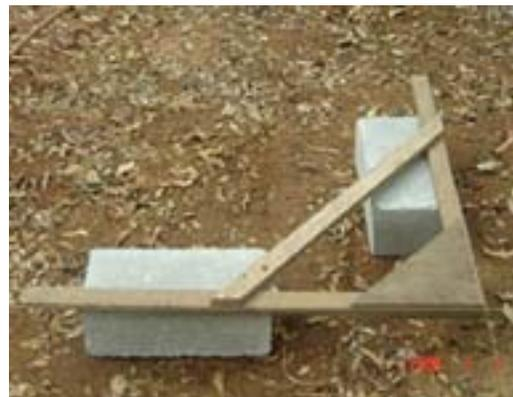
Picture 8: using 3-4-5 method to fix the corners of the building
