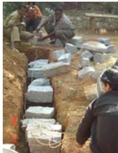
Picture 9: Levelling by transparent water pipe
