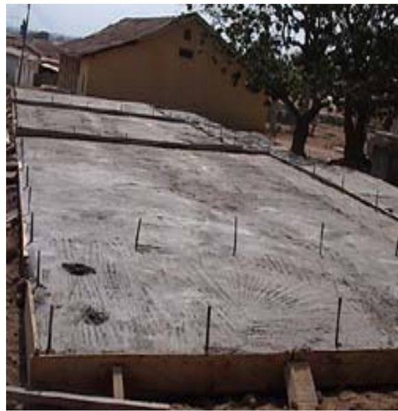
Picture 11-12: Foundation column and ground slab
