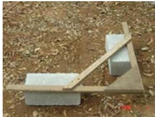
Picture 8: using 3-4-5 method to fix the corners of the building
