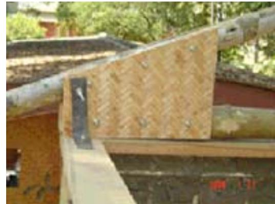
Pictures 25-26: Truss hanging and fixing
