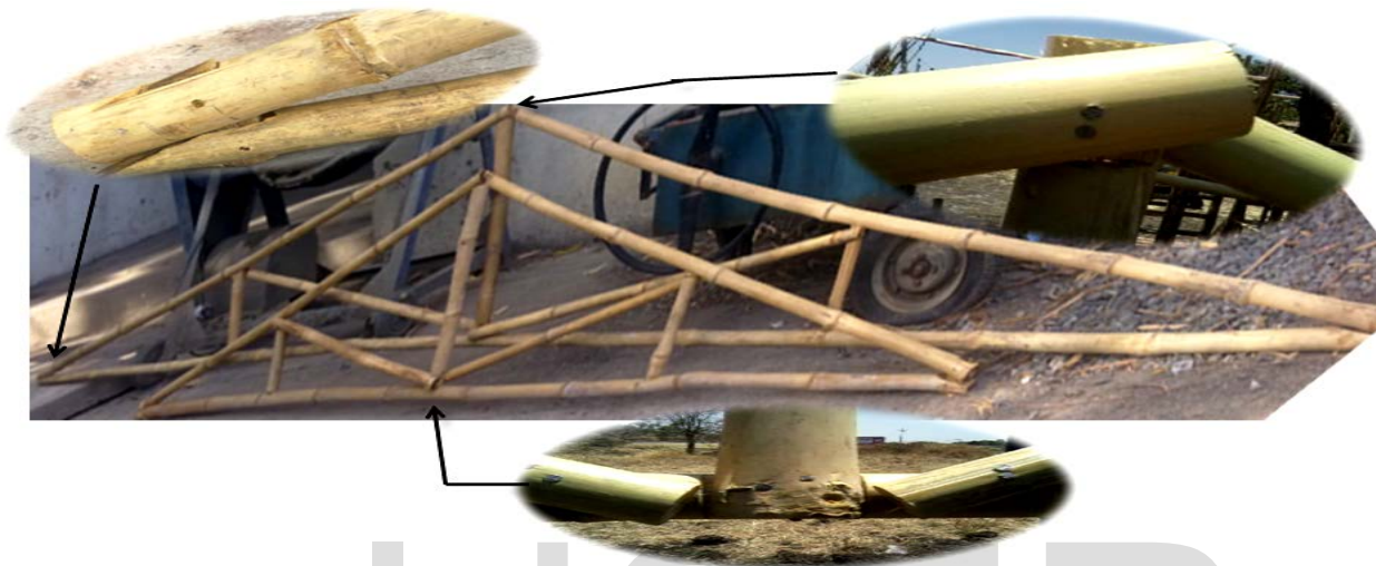
Figure 2.2 Prepared truss at RIT, Rajaramnagar
