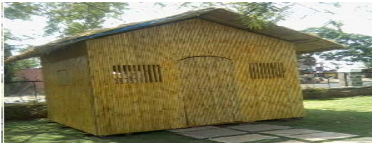
Figure 2.3 Developed roofing system in RIT, Rajaramnagar
