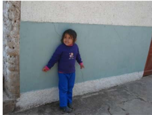
Figure 1: Girl in a place of risk from the damaged building, Peru. Photo: Soluciones Prácticas.
