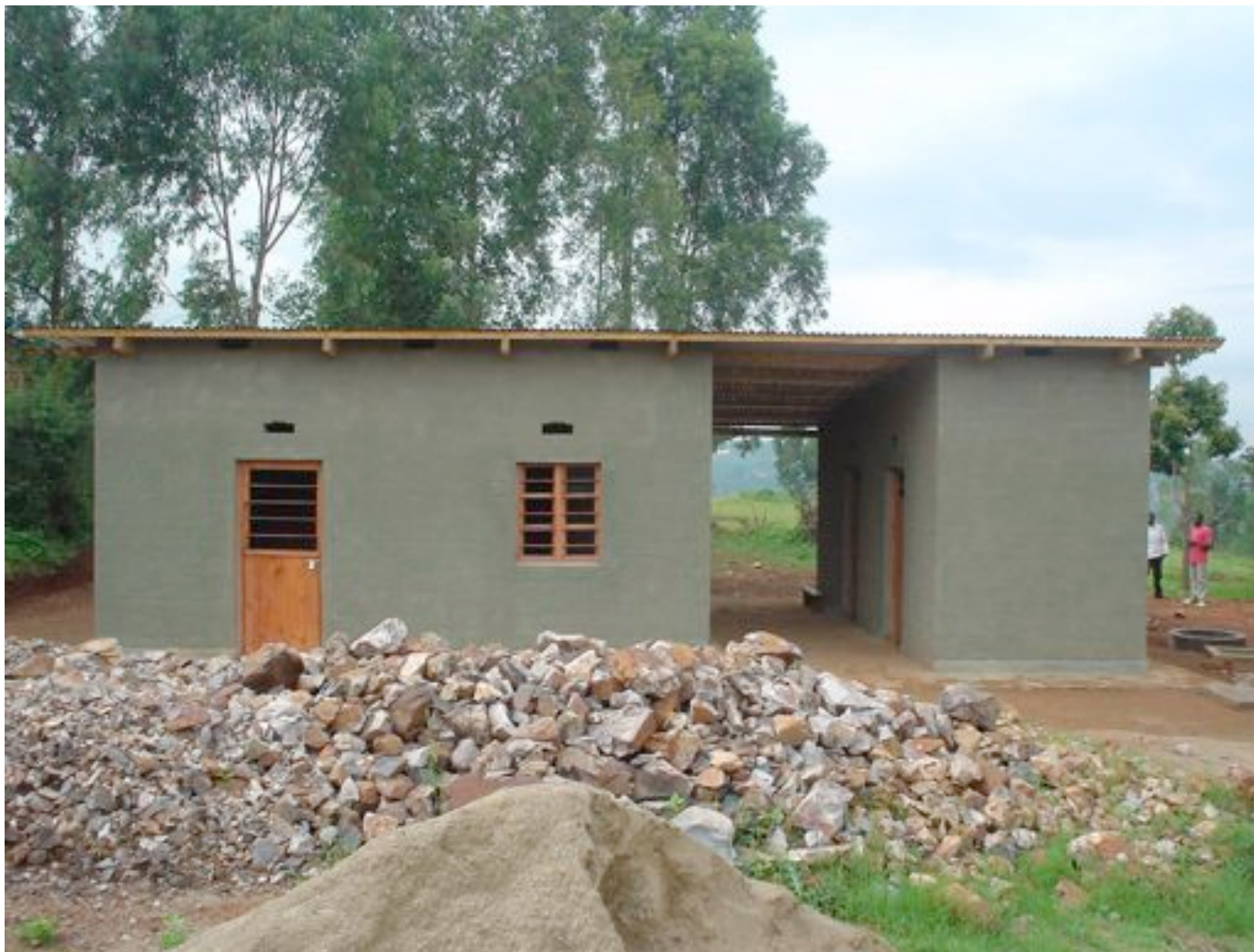
The Model House near completion / Iyi ni inzu –ntangarugero iri hafi yo kuzura.
