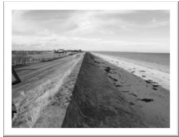
FIGURE 2: DIGUE DE FRONT DE MER
