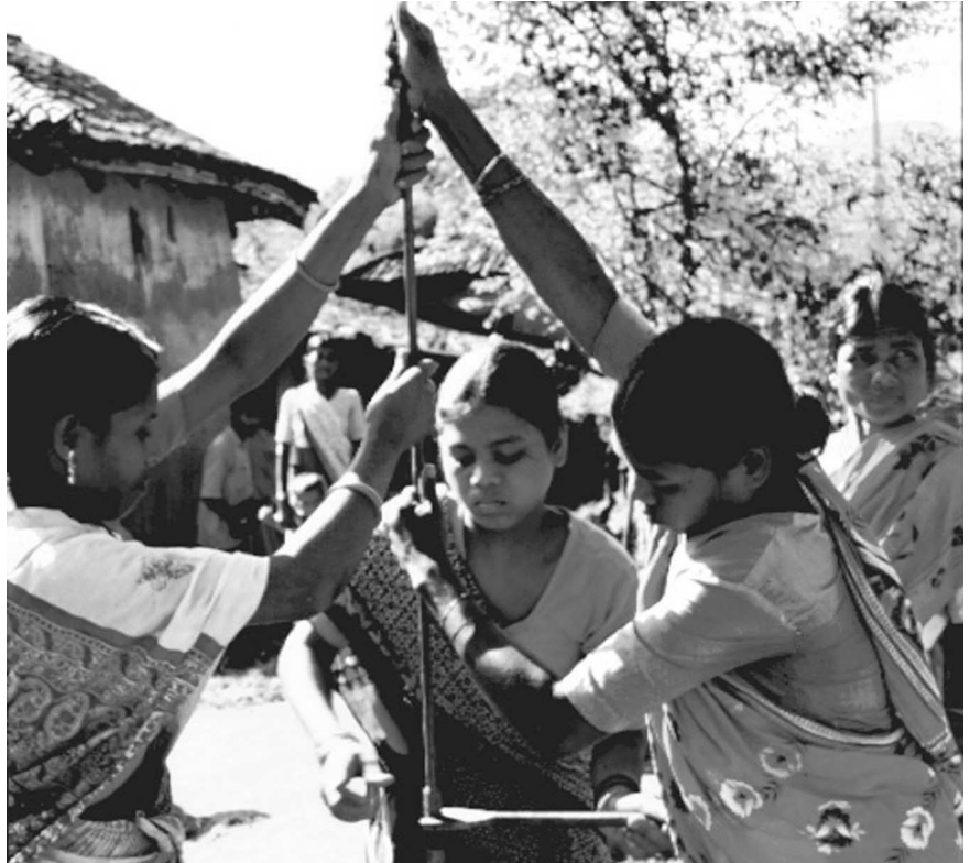
Women mechanics work together to repair a local handpump.
