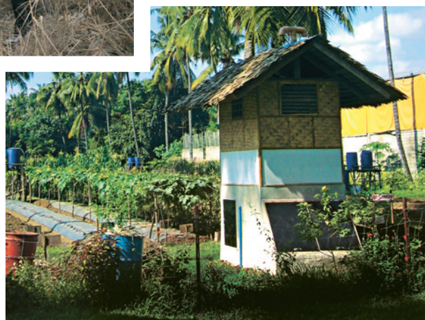
Picture below: UDD toilet provides fertiliser for allotment garden in Cagayan de Oro City (Philippines)
