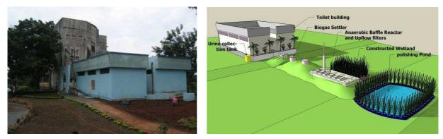
**Fig 3.** Low-flush pour-flush urine diversion toilets at Adarsh Vidya Mandir school (source: ESF). Left: New toilet centre in 2008; right: technical drawing of sanitation system of the school.
