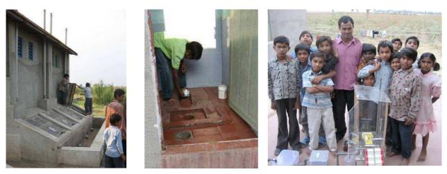
**Fig 2.** UDDTs at the sanitation facility of the primary school at Rayka village. Left: Faeces dehydration chambers with vent pipes; middle: faeces are sprinkled with dry material, e.g. ash/rice husk; right: 'Young scientists' who received first prize for the ecosan school toilet model (source: ESF).
