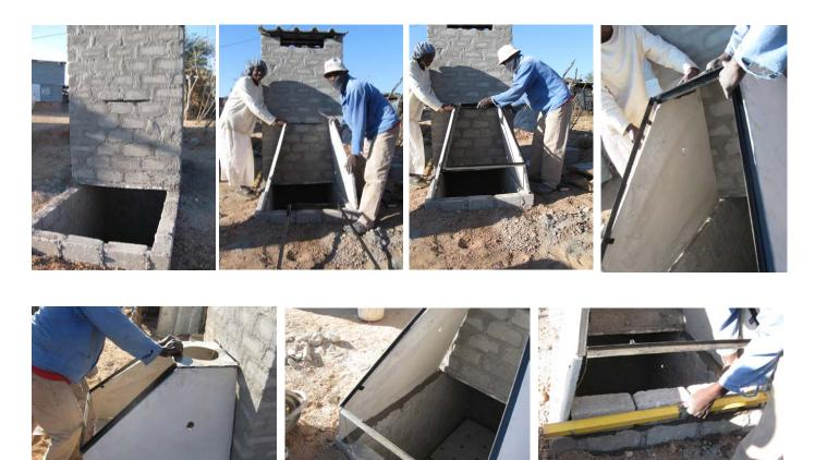
Put the ventilation pipe over the hole on the top of the lid box. Fix it with wire at the roof structure and use the silicon to seal it on the lid box to make it air– and waterproof. Seal as well small gaps between lid box and side plates to prevent any air circulation at the box. Big gaps you have closed with mortar.
