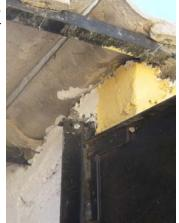
As the floor plate does not cover the whole inside space, add a 100 mm cement slap.
