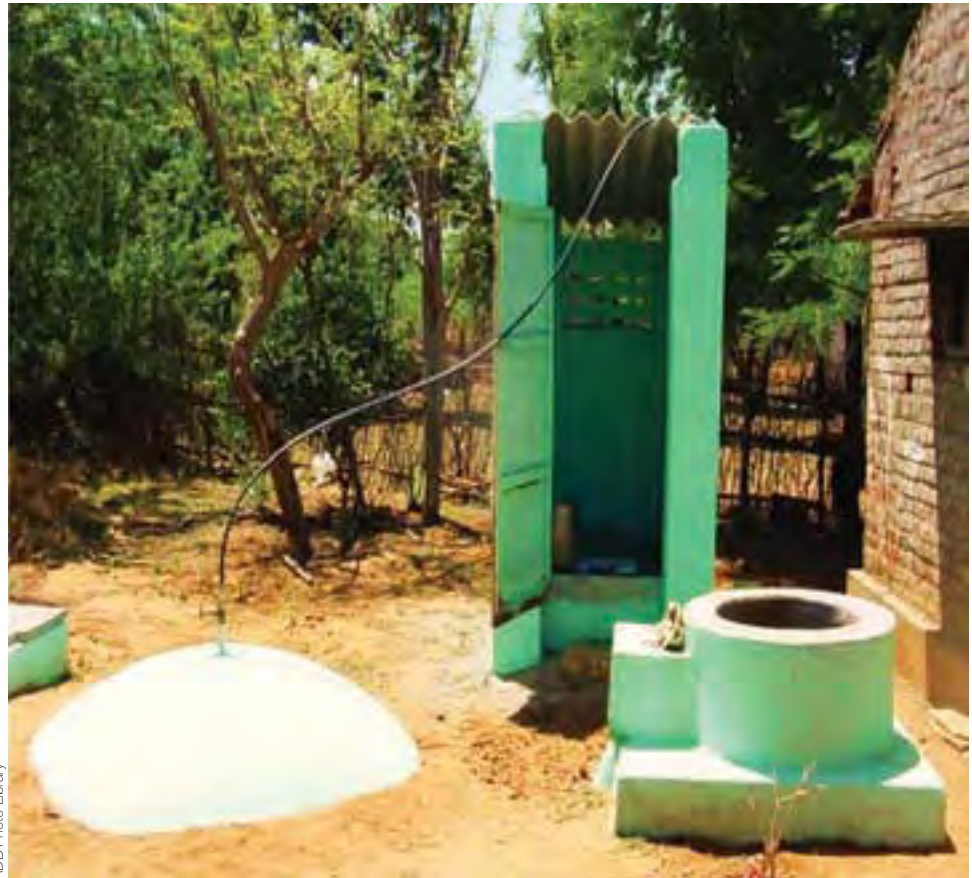
Provision of toilets connected to biogas digesters has helped communities gain access to sanitation and an inexpensive energy source
