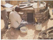
The vaults are constructed off the ground. The slab is placed on the vaults. When the vaults are off the ground, the rain cannot inundate them and the sun can heat the walls and help drying out the faeces.
