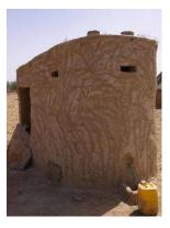
Different types of superstructure are possible, in straw or adobe for example. The roof is necessary to keep the vaults dry and to minimize the access to flies.
