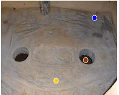
The urine separation on the slab can be done in different ways. The anal cleansing water is drained separately from the cabin.
