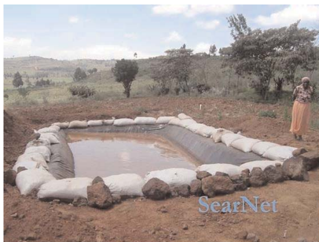
Plastic lining anchored with sand-bags (Image: SearNet)
