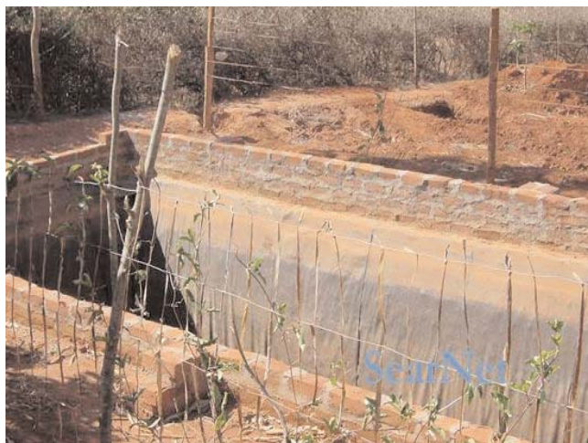
Plastic lining anchored with brick wall (Image: SearNet)
