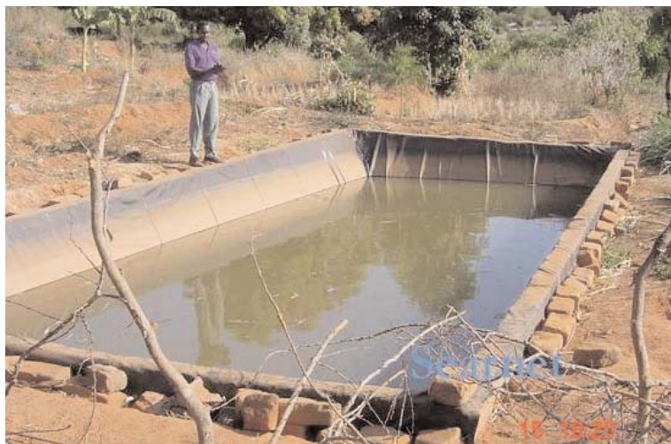
Plastic lined tank (Image: SearNet)
