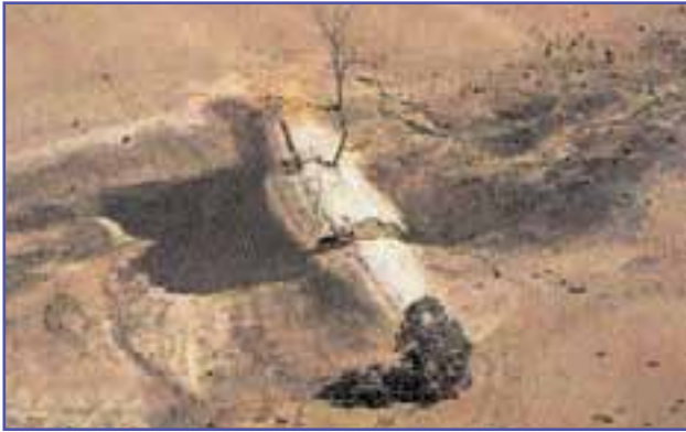
Small earth dam, broken due to lack of a sufficient spillway. Photo from booklet on water harvesting by the State Department in Western Australia.
