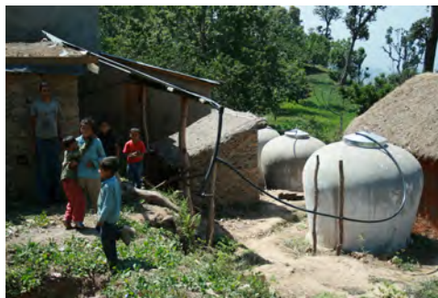
Figure 1. Rainwater harvesting tanks in Bubeyrakhe, Nepal (photo: RAIN)
