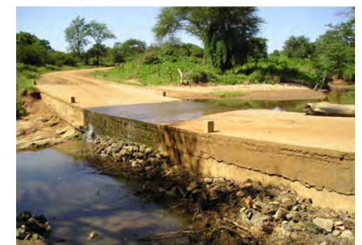
Figure 3 : Irish bridge (Source : Nissen-Petersen, E, 2006)
