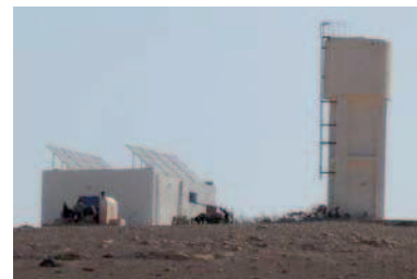
Figure 22. Fresh water tank, building and PV field.
