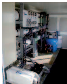
Figure 28. SWRO desalination plant. Container housing SWRO unit.
