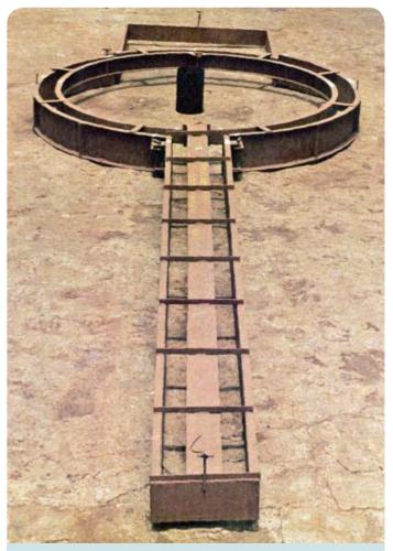
Fig. 2.53 Mould for the platform, Tanzania
