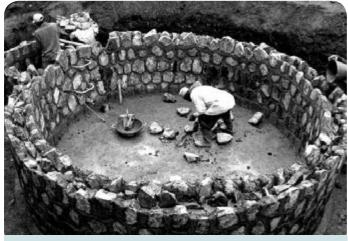
Fig. 4.27 Masonry groundwater tank, Lesotho
