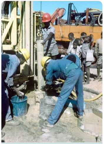
Fig. 2.43 Placing the gravel pack, Zambia
