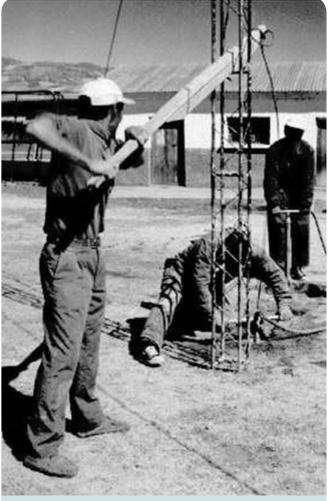
Fig. 2.31 EMAS drilling
