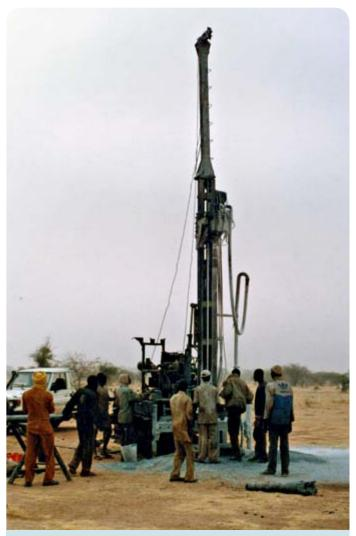
Fig. 2.10 Rotary drilling, Ethiopia
