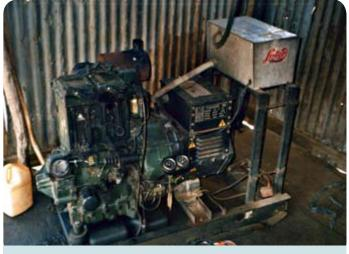
Fig. 4.17 Generator for submersible pump, Eritrea © Skat
