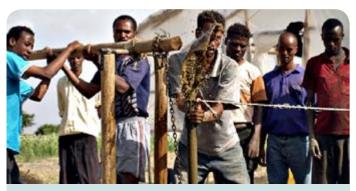
Fig. 2.26 Rota sludge drilling
