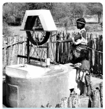
Fig. 1.14 Nicaragua rope pump
