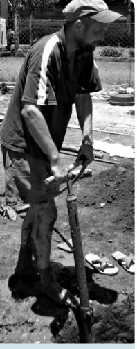
Fig. 2.33 Hand-operated mud pump
