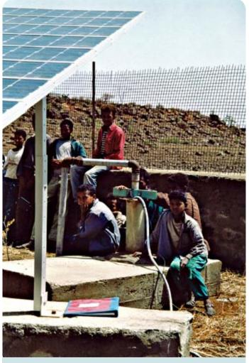
Fig. 3.11 Solar pumping system
