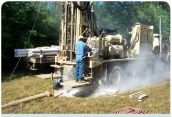
Fig. 2.11 Down-the-hole hammer drilling
