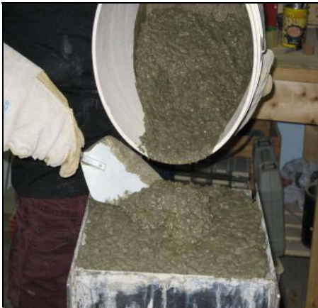
Step 7 - Fill the mold full of concrete
