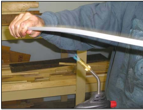
If the polyethylene tubing is stiff, it may need to be heated in order to bend it
