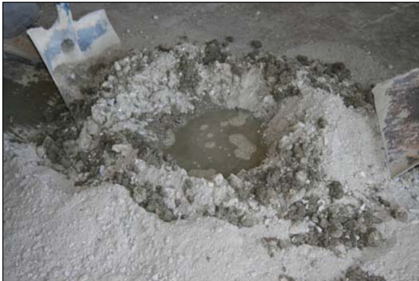
Mix the dry ingredients together using a shovel. Make a shallow hole in the centre and pour water into the hole. Mix thoroughly and continue to add water until it reaches the proper consistency.
