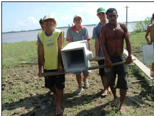
Carrying filters using wood supports
