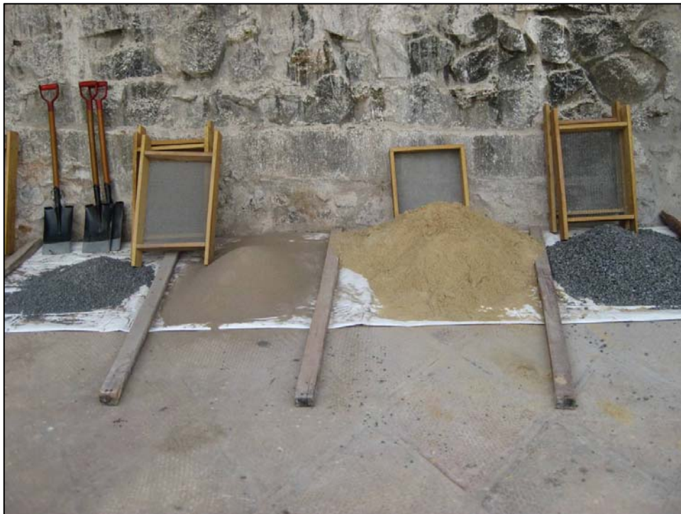
Tidy and separate piles will keep the sand and gravel from mixing together
