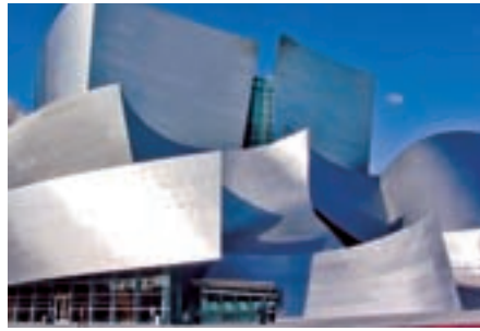
Cost and time savings resulted during various phases of design and construction of the Walt Disney Concert Hall in Los Angeles, above, because of cooperation among all parties involved, according to one of the industry presenters at the WSU symposium. (Photo courtesy of M.A. Mortenson Company)
