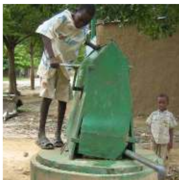
Rope pump, Sabangali quater, N'Djamena
