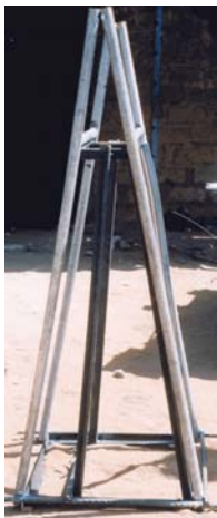
structure in jig
