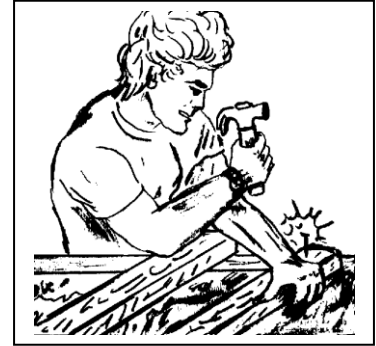
c.1.5. Beams nailed on the wellhead
