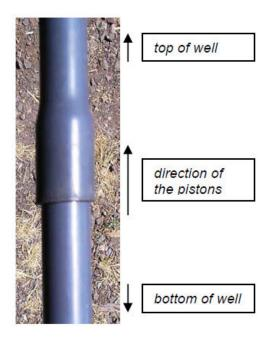
Make sure during installation all connections are constructed with the male parts towards the bottom side of the well and the female parts towards the top side of the well.
