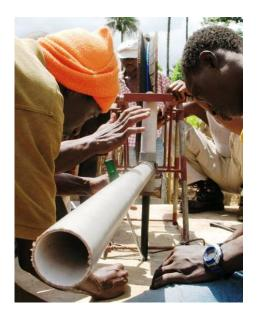
Once you have fixed the security rope. Place some small stone between the PVC pipe and the cement inside the hole. Then seal the hole with cement. Let it dry
