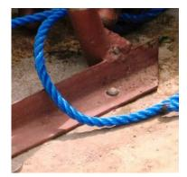
3) If the bolt is to short to fix the nut, use a hammer and a chisel (or at least a screwdriver flat) to brake thin layers of the cement by mortising slowly the surface around the bold
