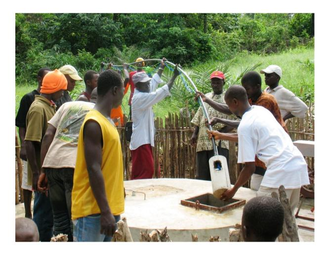
Don't turn the pipe around during installation to prevent the rope from winding around the pipe. Lower it straight. Keep the rope on one side of the pipe.
