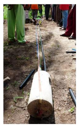
4) Use a second nylon rope without knots or piston. Tie it to the upper hook of the guide box between the inlet and outlet Pipes. This security rope will be useful to lower the pump inside the well or to hold it out of the well for reparation.
