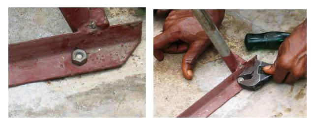
5) Finally, fix the front of the frame to the iron rod of the cover. Fix it with biding wires;
