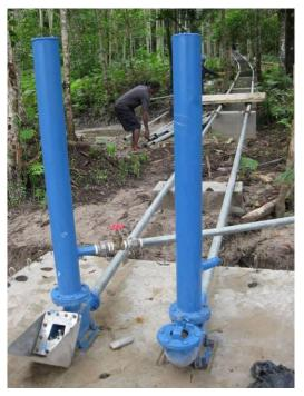
Figure 23: Drive pipes and supports
