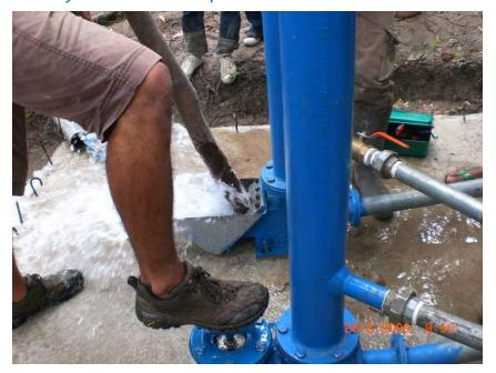
Figure 26: Priming the Hydraulic Ram Pump
