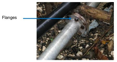
Figure 6: Drive pipe and flanges
