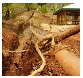
Figure 21: Burring delivery pipe
