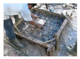
Figure 7: Construction of pump basement, NTT
