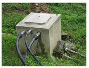
Figure 5.a: Header tank for 6 pumps from AID Foundation Figure 5.b: Header tank for 2 pumps from AID Foundation
