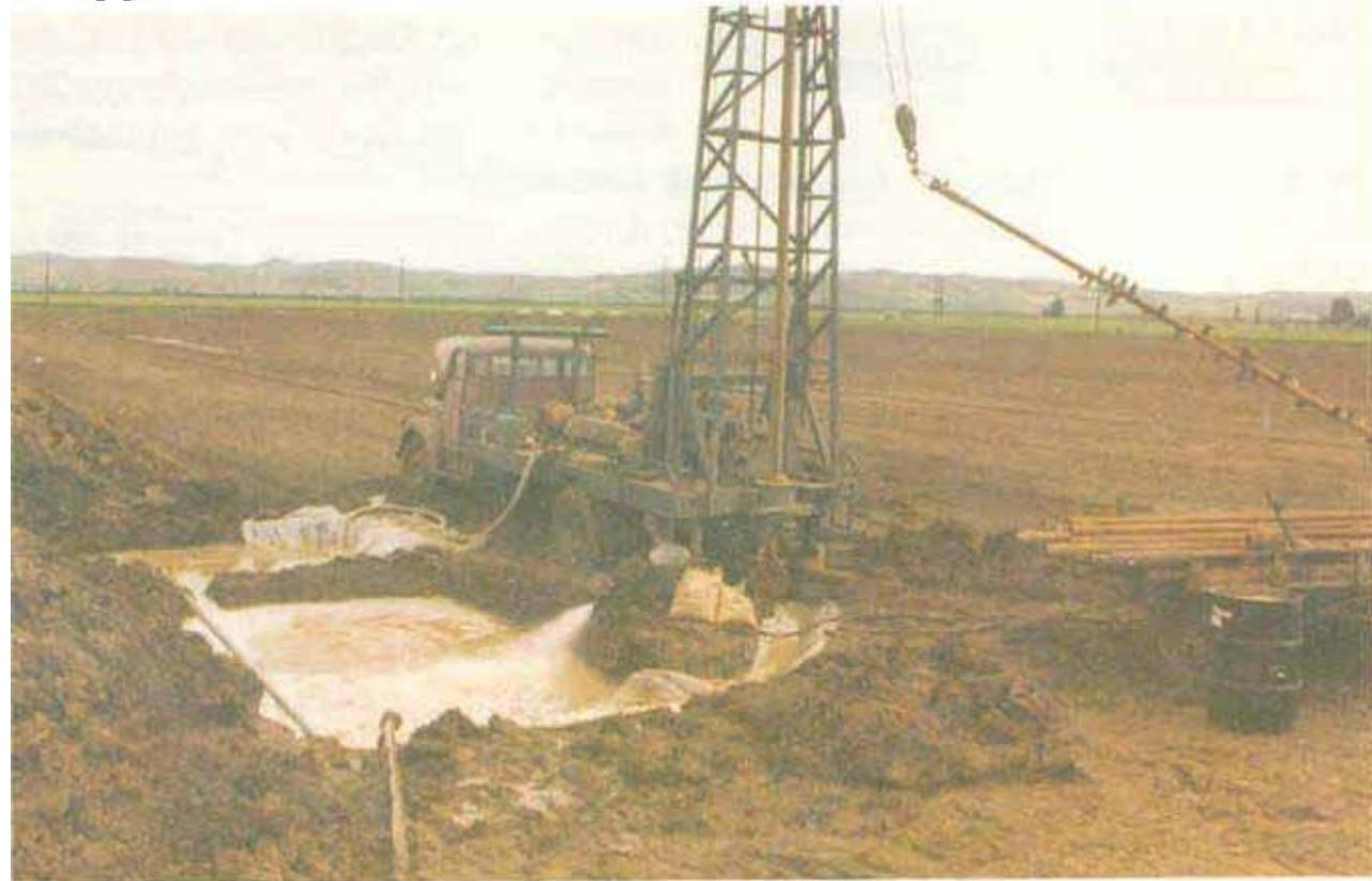
**Figure 6.3:** Drilling fluid from the borehole flows into the larger pit where the cuttings settle out.
