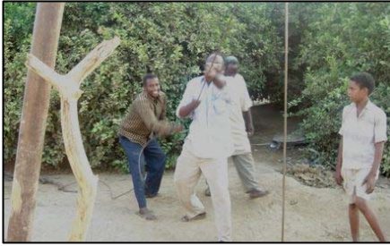
Pic 5: People pulling up the jardel full of mud from the bottom of the well
