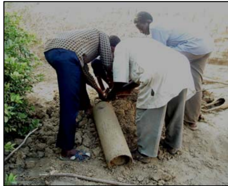
Pic 1: Workers attach the Bailer tool
