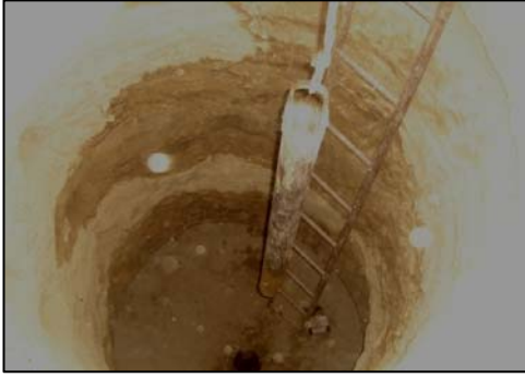
Pic 2: The Bailer tool is lowered into the well hole
