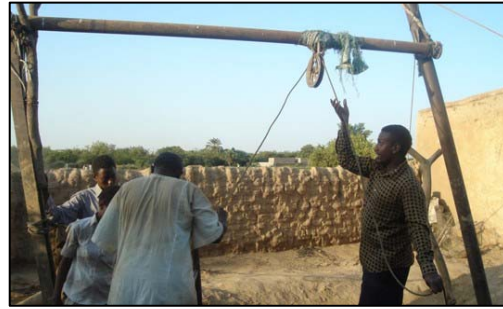
Pic 4: The rope from the winch is tied to the jardel.
