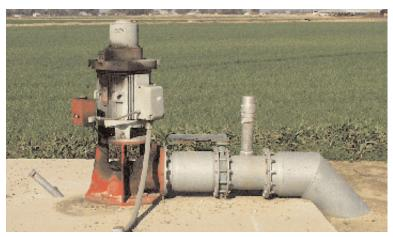
Figure 3. Properly completed well with elevated concrete seal (but with leaking lubricant).
