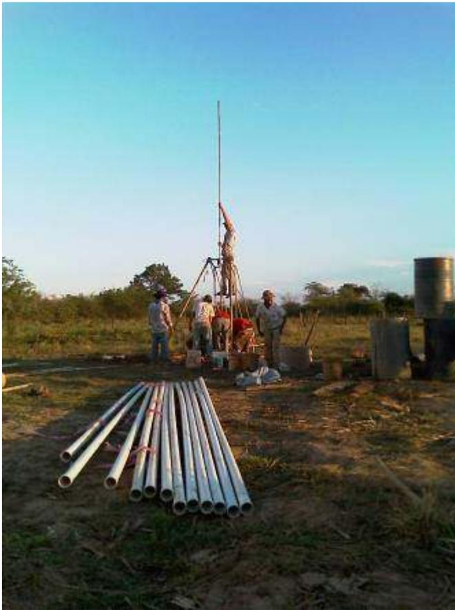
Casing laid out and ready to case well open hole dug well. . Each casing length is 6 meters. Notice prepared filter on left. There are 12, 6 meter tubes class 9 pvc. Casing pipes that were placed in this well. . The well was 69 meters deep.
