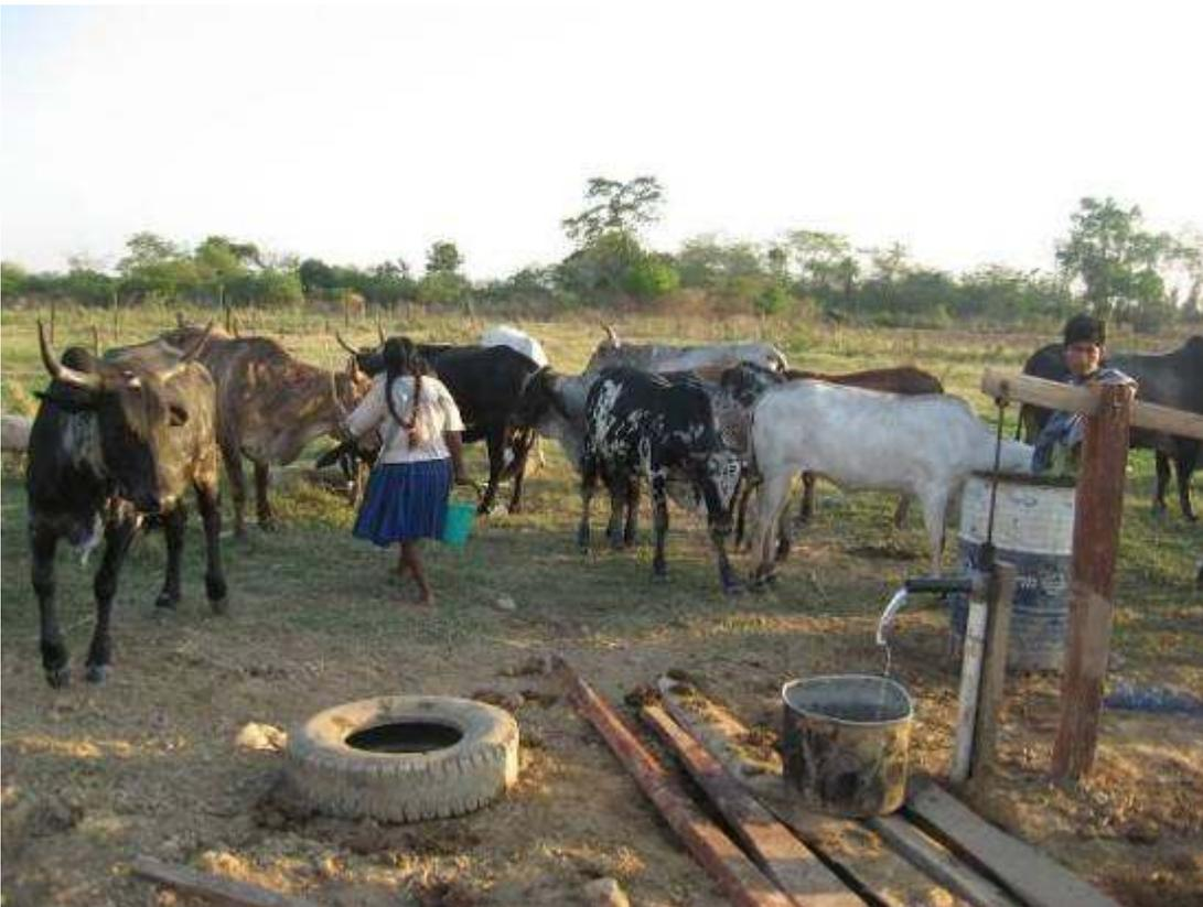
Initial pump set up so user can water cattle. . column and pad added later but not shown. Bentonite plugged seal and grouting.
