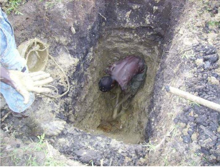
Recovering a drill bit during trial drill Rabondo Kenya May 2006 after passing through hard shallow lithified layer.
