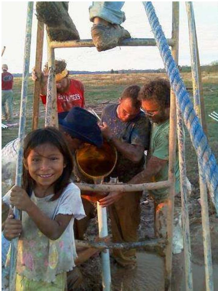
Cased well, Water being poured in casing to counter weight buoyancy of casing against 69 meters of bentonite water drill mud.
