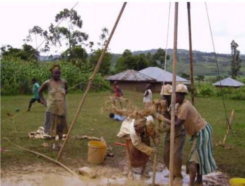
Penetrating hard laterite layer in Rabondo Kenya. Two wells drilled in one week trial drilling trip 2006.
