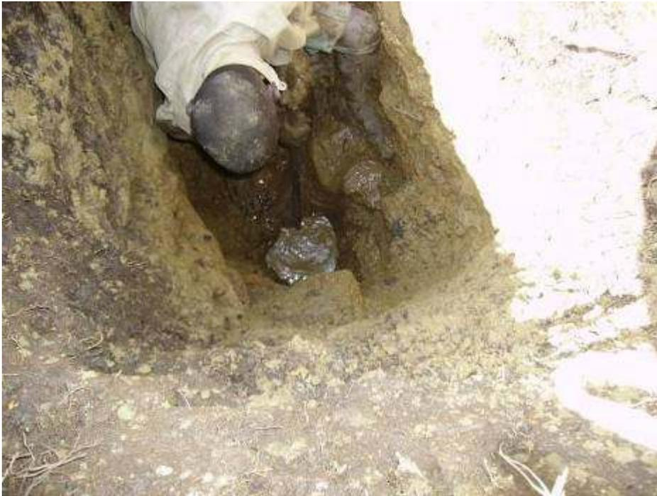
Worker digging with iron rock bar to penetrate hard rock layer.
