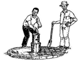
Place reinforcing wire and a mold for the hole.
