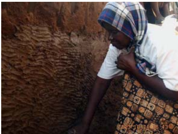
Picture 3: Tank lining/ Plastering ©Practical Action/Douglas Gumbo
