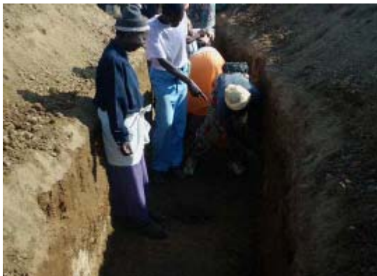
Picture 1: Foundation of the underground tank ©Practical Action/Douglas Gumbo
