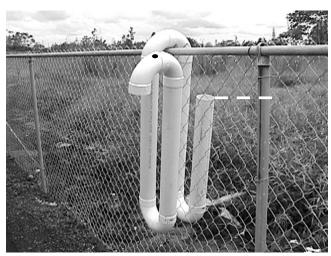
An overflow device that will keep the water level as indicated. The pipes on the near side of the fence hang outside the tank. In this design, a hole must be made on the top of the pipe in the foreground for the system to function properly. If a T joint is used instead of an elbow, the hole is not needed.
