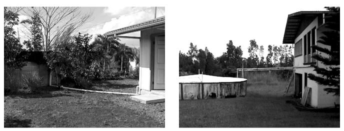
The U-shaped downspout-to-tank configuration at left is typical but undesirable. The pipe runs down from the roof, across the ground, then up and over the tank. Between rains, water is left standing in the pipe. In the system at right, the downspout is completely drained by gravity.
