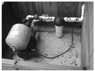
A small but typical electric pump. The pump sits below a pressure chamber. A coarse filter hanging from the inlet pipe filters the water before it enters the house.
