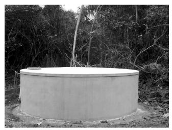
Ferroconcrete tanks, also known as ferrocement tanks, are new to the local market and growing in popularity. Like solid concrete tanks, they can be designed into a home's structure.
