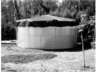
Pipe arches supporting a mesh cover keep it from sagging into the water.
