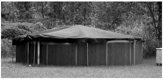
A large swimming pool tank with pipe arches holding up a mesh cover. These tanks are popular for their price and ease of assembly.
