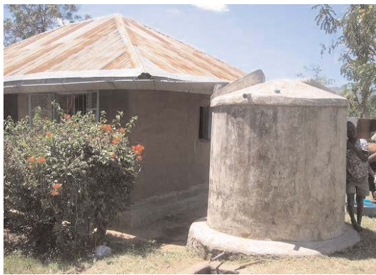
Roofwater tank (Image: Sarah Watson, PACE)
