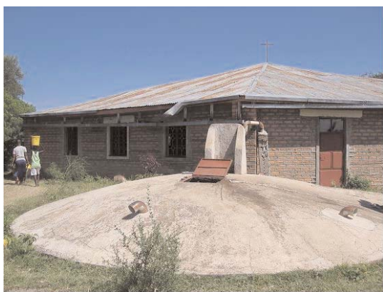
Roofwater cistern (Image: PACE)
