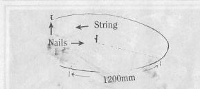
On a flat surface draw a circle the diameter of the tank you want to build.
