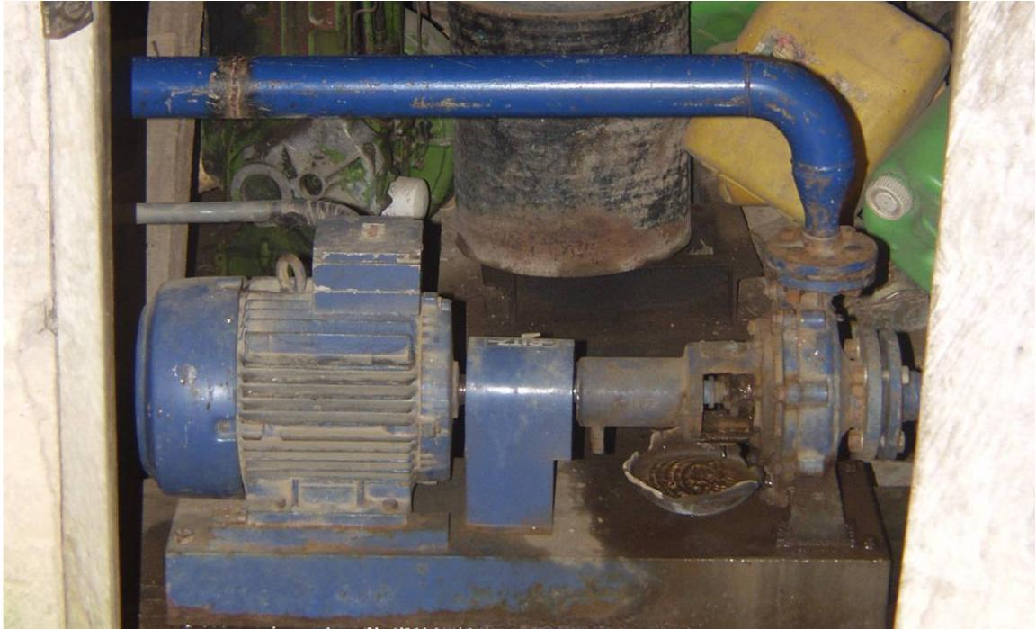
Figure 41: Centrifugal pump driven by electric motor in Maase-Offinso, Ghana.
