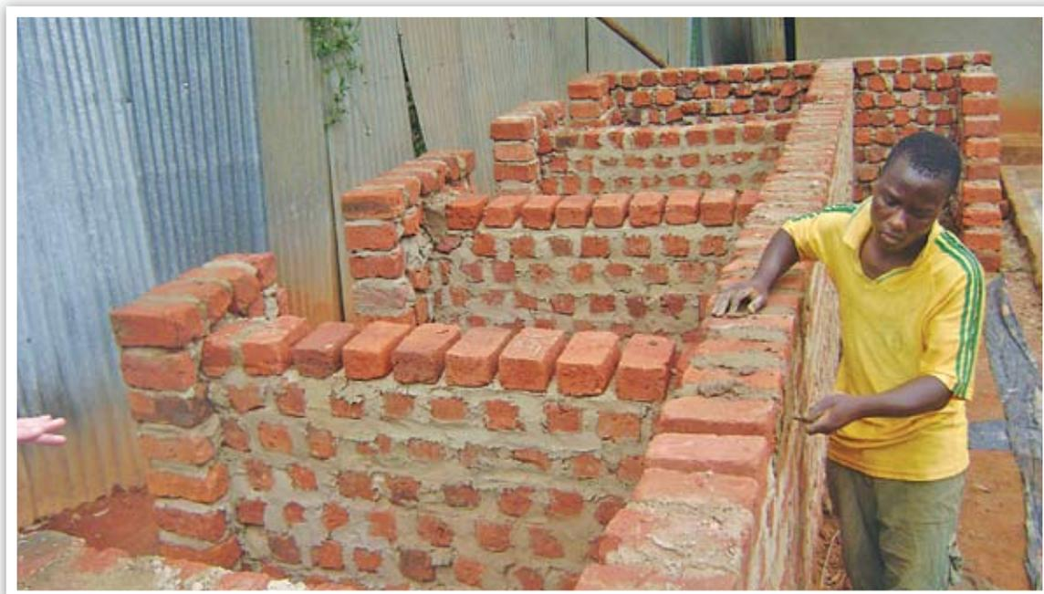
*Constructing a brick chamber for an ecological sanitation toilet at Ggaba PTC*
