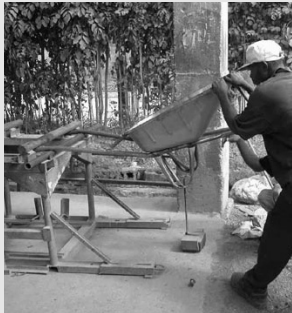
Figure 20: Cintrage du tube principal
