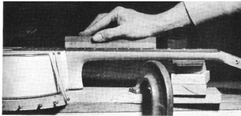
Fig. 101 Leveling frets with carborundum stone
