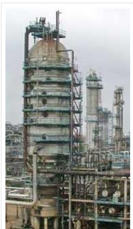
Large-scale, industrial vacuum distillation column [15]
