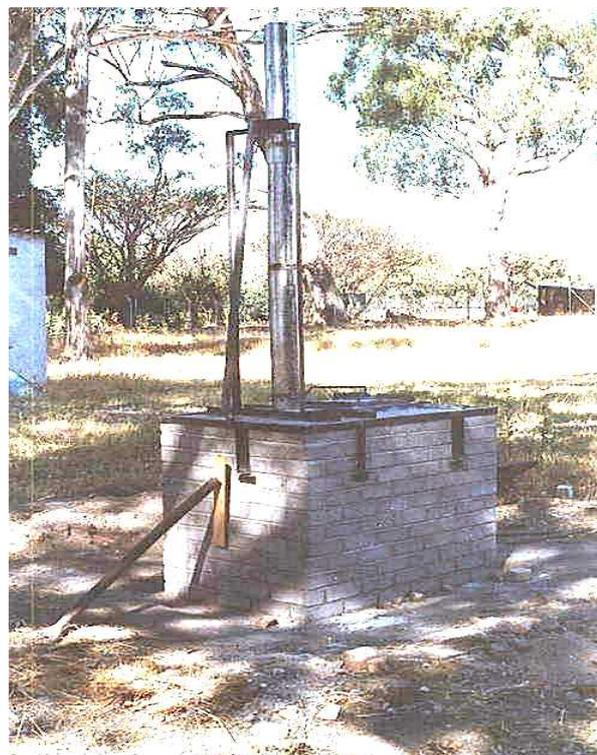
Figure 11: Stack support frame
