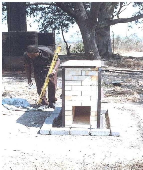
While building up the outer wall, the ash door and air inlet tubes should be fitted. Where they pass into the combustion chamber they should be fixed in position using fire cement.
