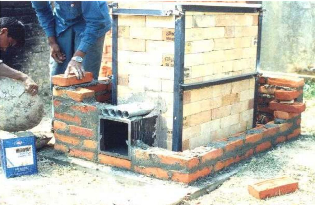
Figure 6: Air inlet pipes and ash door
