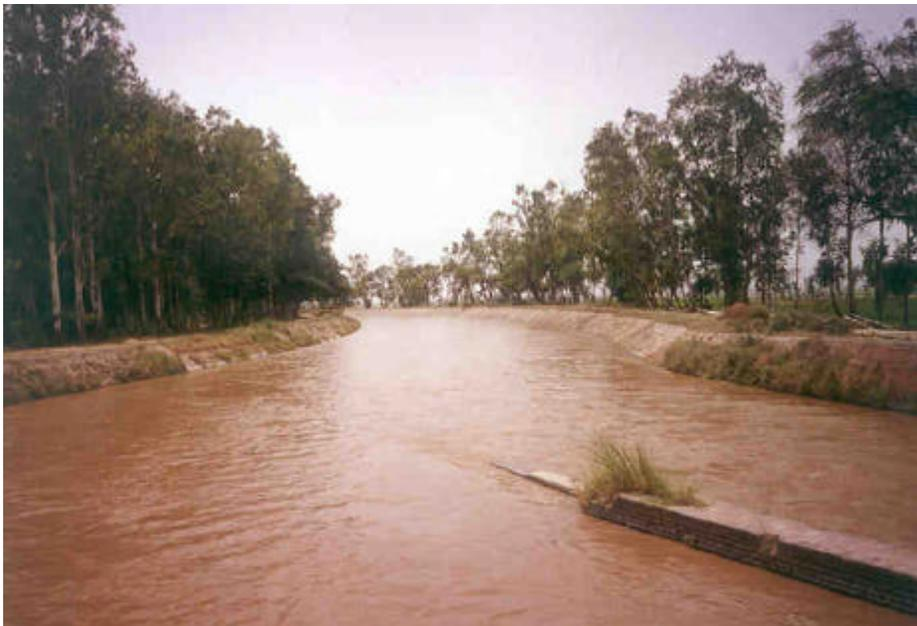
Fig.14. Movement of turbid water reduces the growth of submerged aquatic weeds
