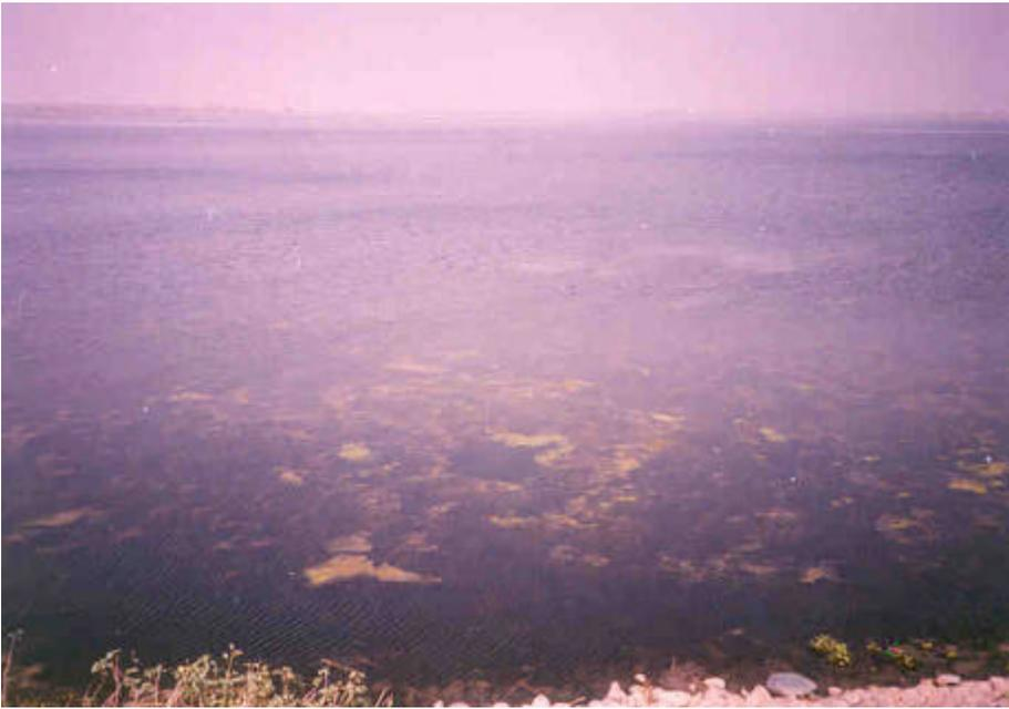
Fig.16. Earthen bank large reservoirs having shallow depth near banks encourages the growth of submerged aquatic vegetation
