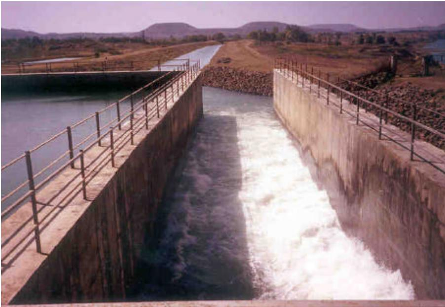
Fig.9. High velocity of water in flow water system discourages weed growth
