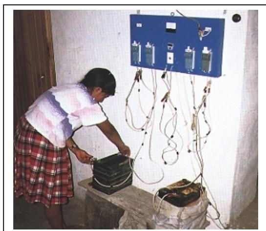
Figure 13-4 Battery charging with hydro power (Peru)
